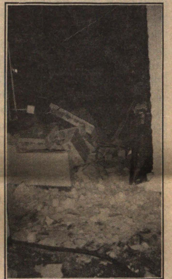
Photo by Katie Oen Locker room demolition began May 22.
